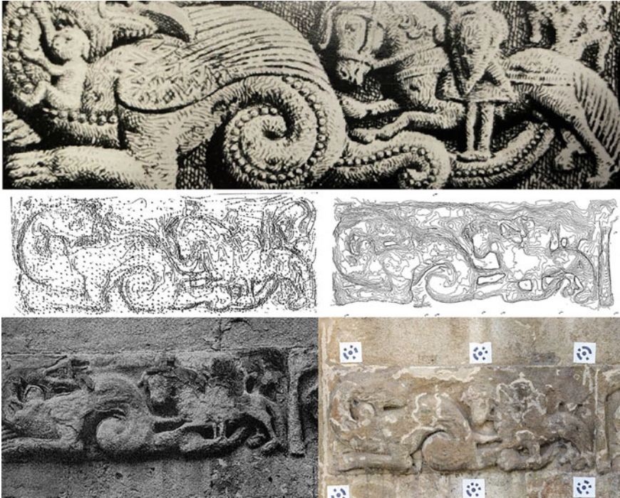
Fig. 4 St. George and the Dragon tile. Above: the historical drawing by F. De Dartein [11]. Centre: Images of the studies conducted by G. Cassinis: topographic points (center left) and isolines (center right). Below: comparison between the mid-1900s photo (left) and the current (right) highlights the severely altered state of conservation
