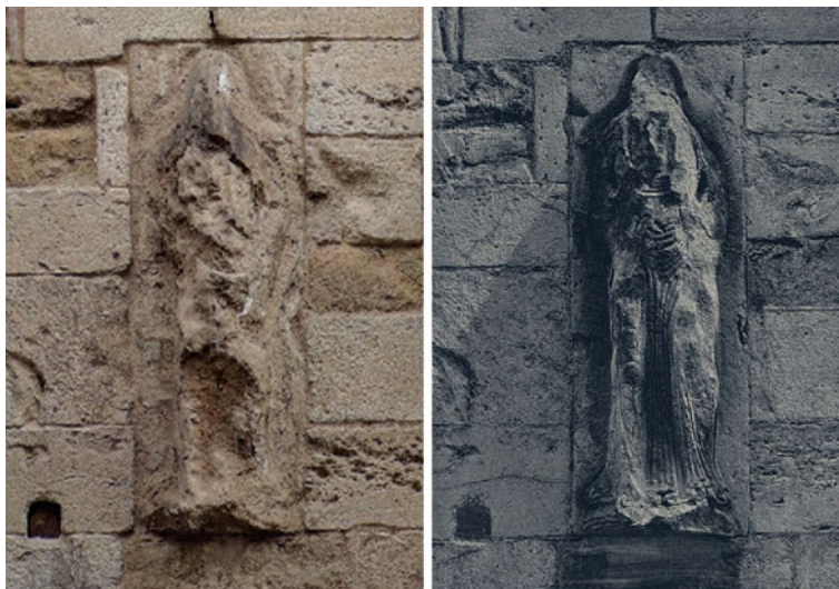
Fig. 2 Comparison between the current status of conservation of a sandstone decoration (on the right) and its state of conservation in 1942 (on the left) thanks to the photographs of the working group of Prof. Gino Cassinis. The historical photograph (on the right) represents the status prior to the restoration carried out in 1963
